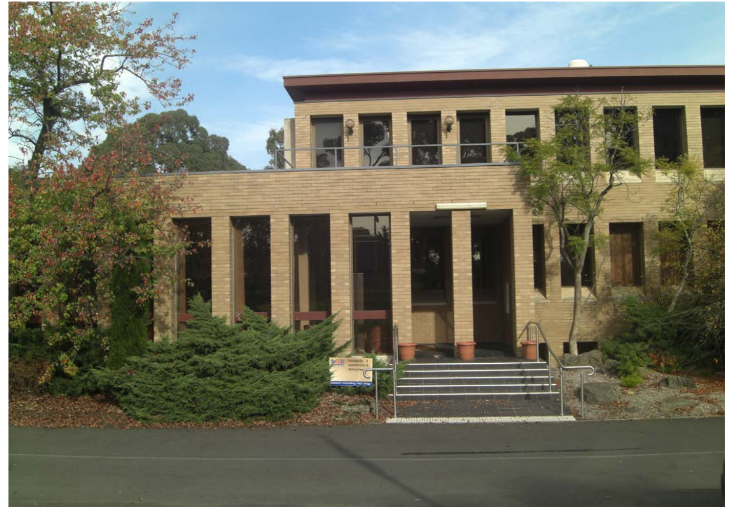
Fig. 36 Existing heritage administration building
