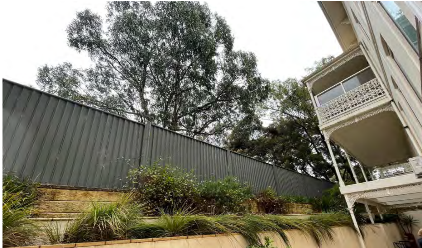
Figure 32. Photo taken from ground floor of Victorian Grange Aged Care building east of Site looking north
