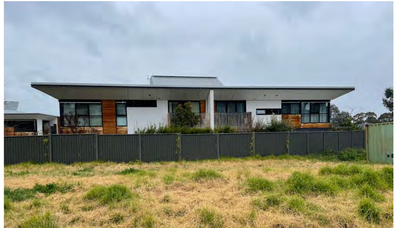
Figure 25. Photo looking south of western most Victorian Grange Aged Care facility
