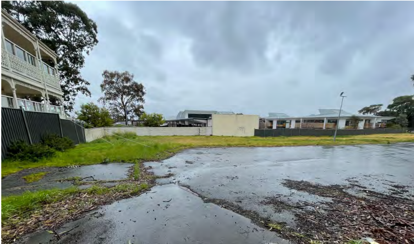
Figure 22. Photo from eastern boundary looking south towards Victoria Grange Aged Care facility
