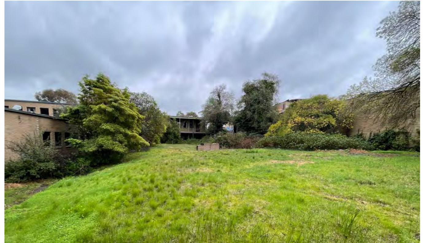
Figure 20. Photo looking north-west towards courtyard and rear of Administration Building
