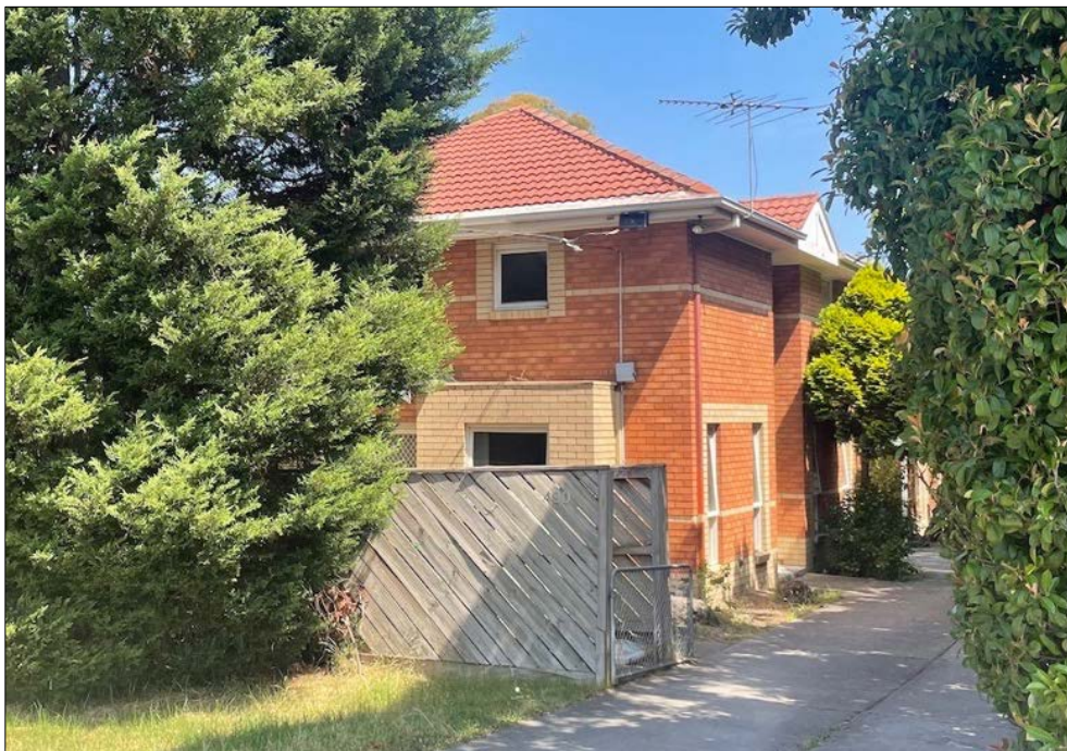
Figure 19 Former ARRB housing in the north-west corner of the site (ie Flats 1 & 2/490-500 Burwood Highway).
