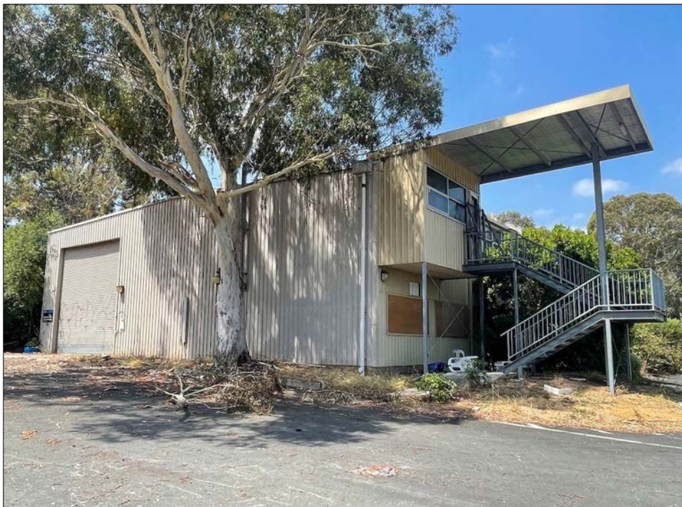
Figure 15 The Truck Bay/Mezzanine.
