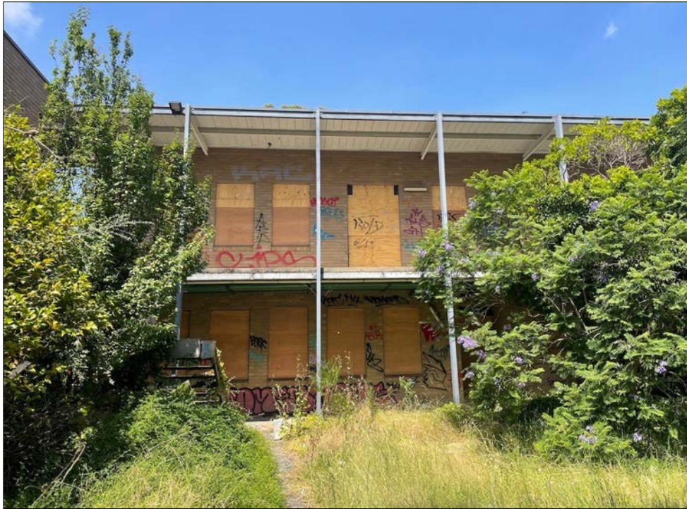
Figure 12 The west elevation of Research Wing 2.
