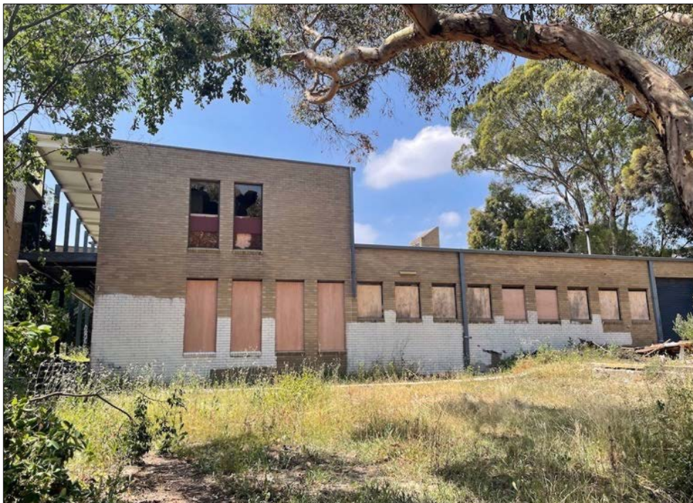
Figure 13 The south elevation of Research Wing 2.
