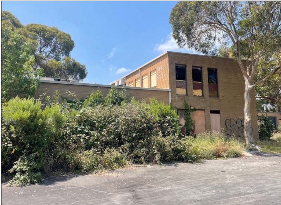
Figure 14 The south elevation of Research Wing 3.
