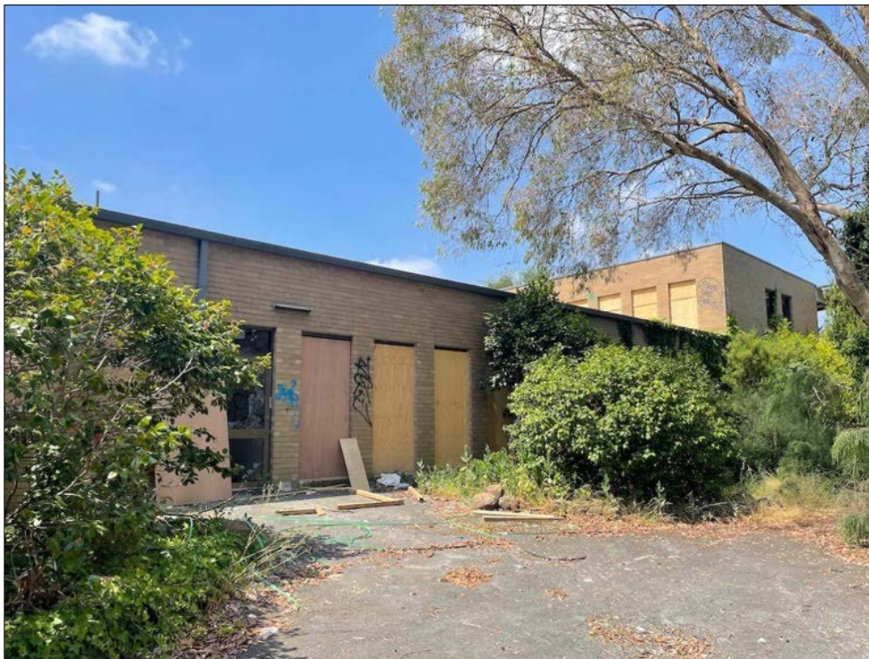
Figure 11 The south elevation of Research Wing 1.
