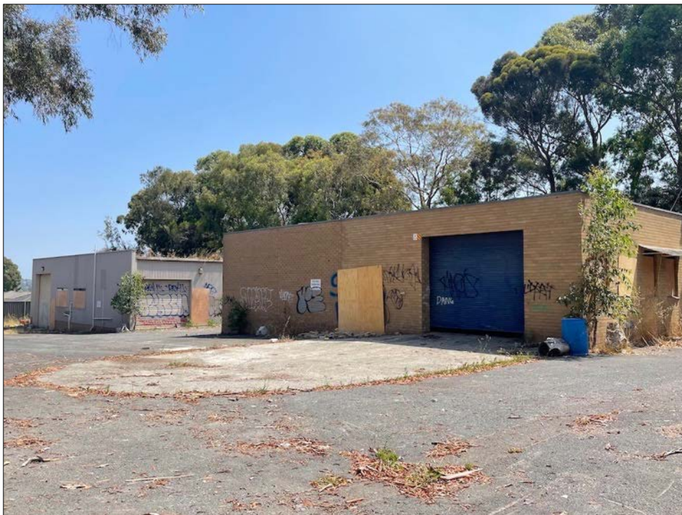
Figure 17 The RMS Lab (foreground) and Concrete Lab/HV workshop.
