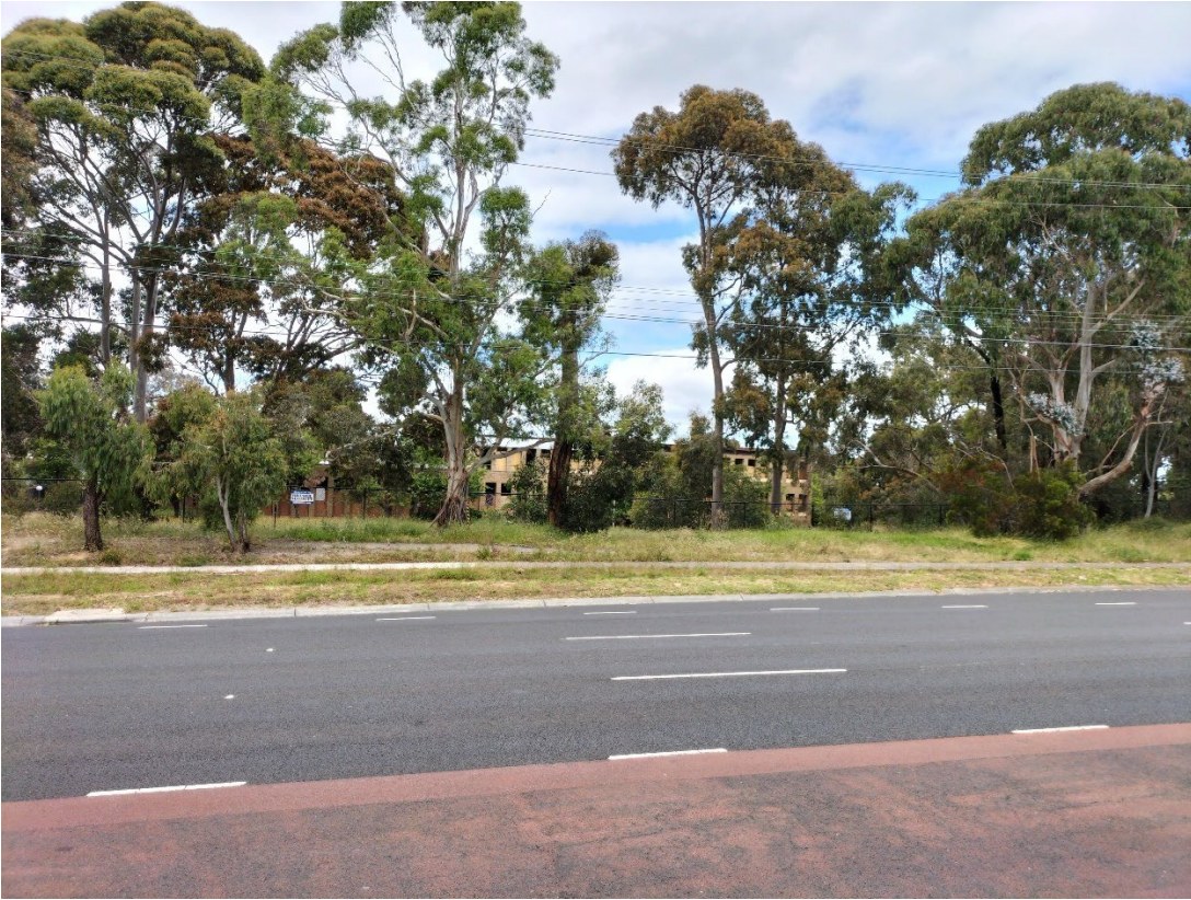
Picture 1: Review site from Burwood Highway
