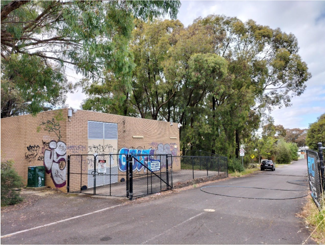
Picture 3: View of site's main entrance and substation
