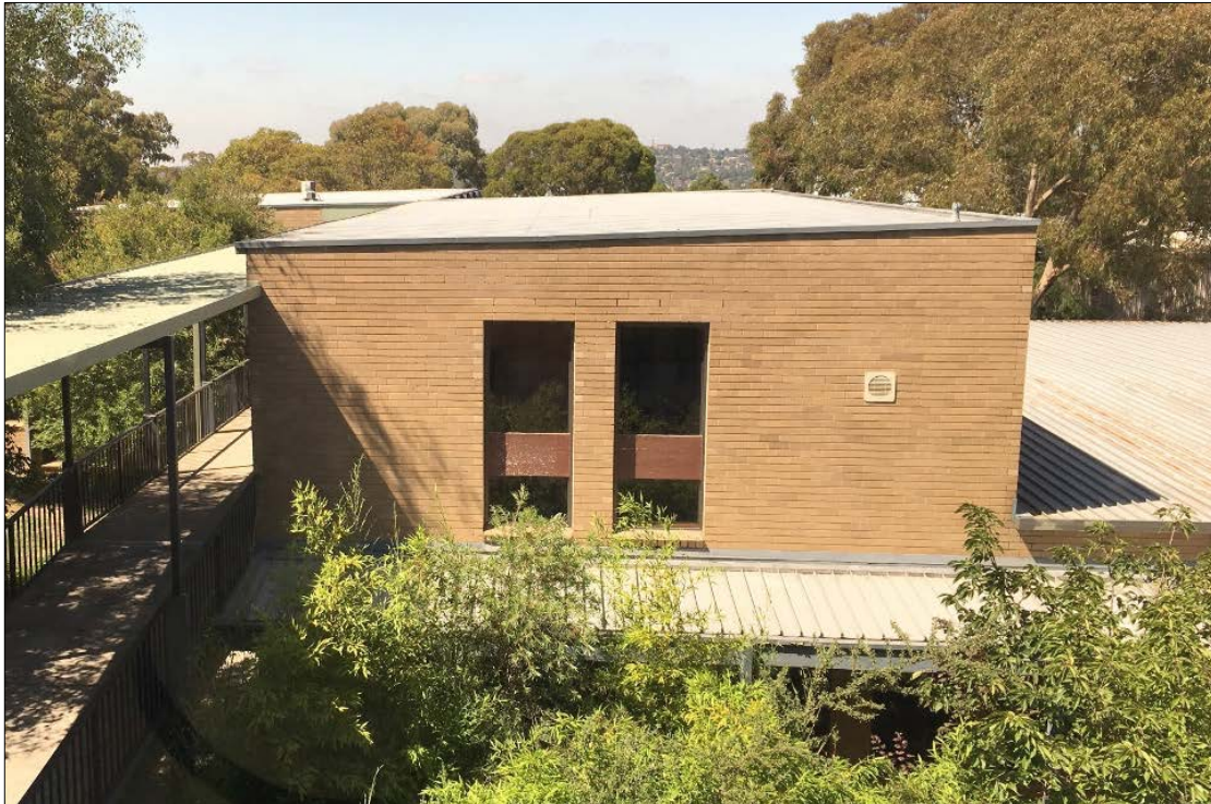
Figure 29 The north elevation of Research Wing 1.
