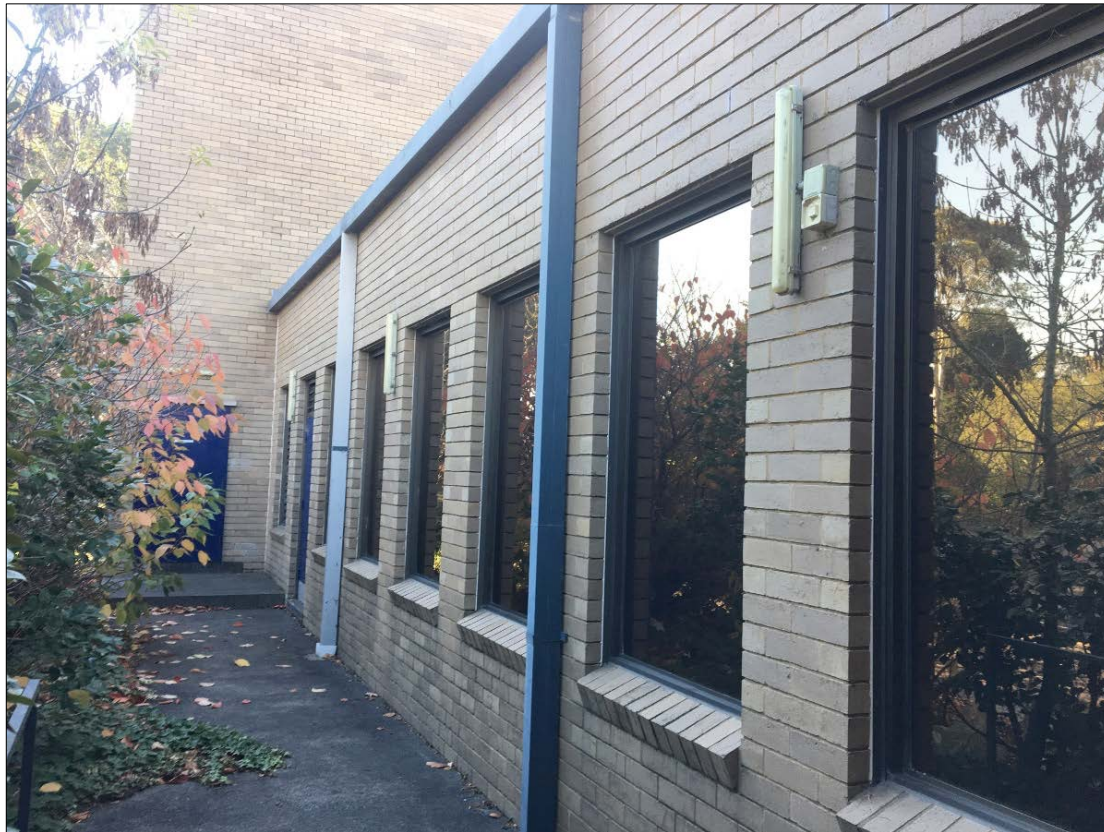
Figure 28 The west elevation of the west wing.
