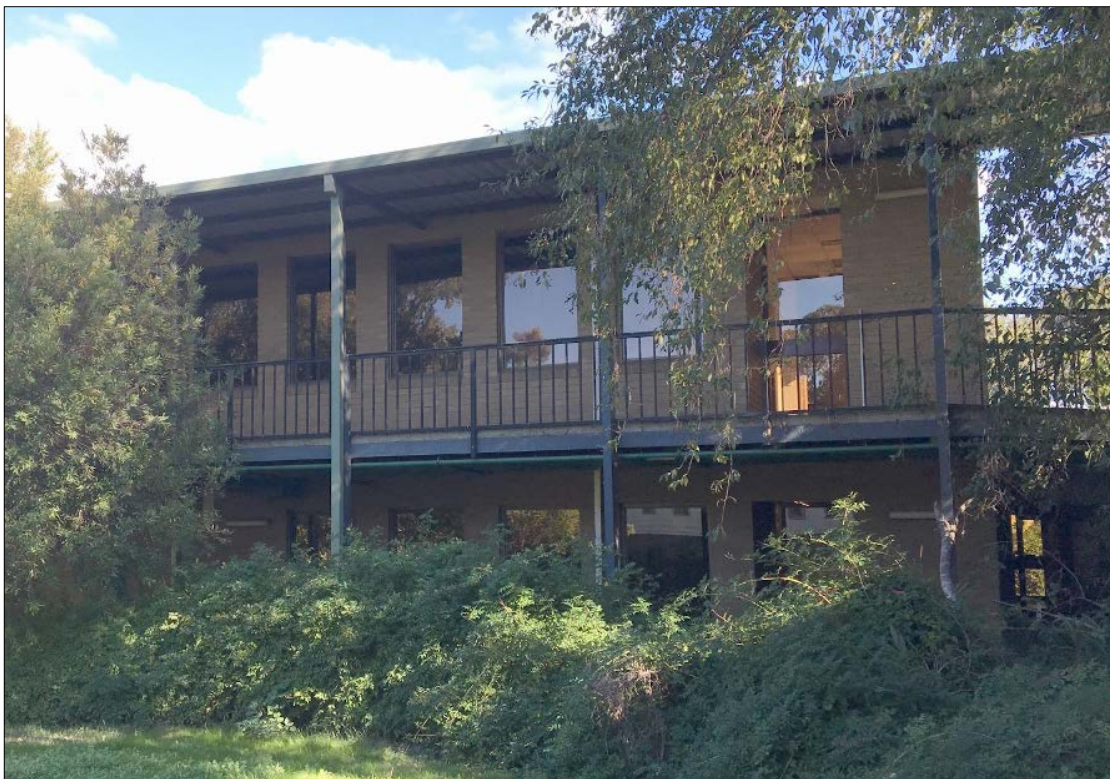
Figure 30 The east elevation of Research Wing 1.
