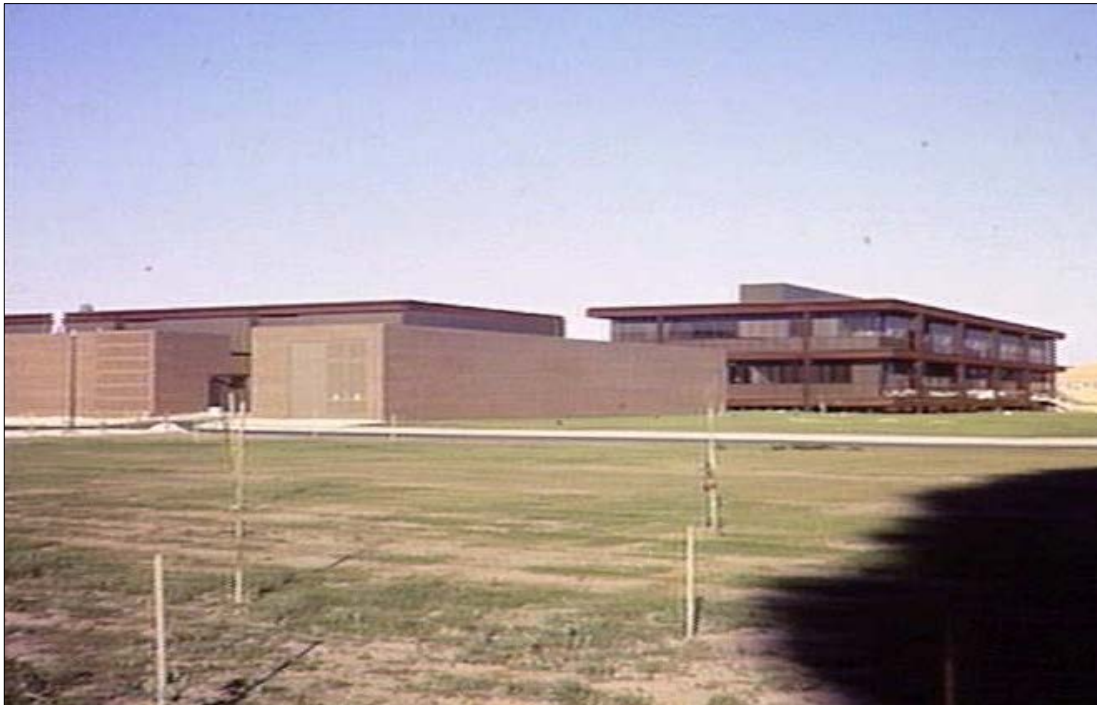
Figure 55 A c1969 photograph of the BHP Research Laboratories, Wellington Road, Mulgrave. Source: State Library of Victoria.
