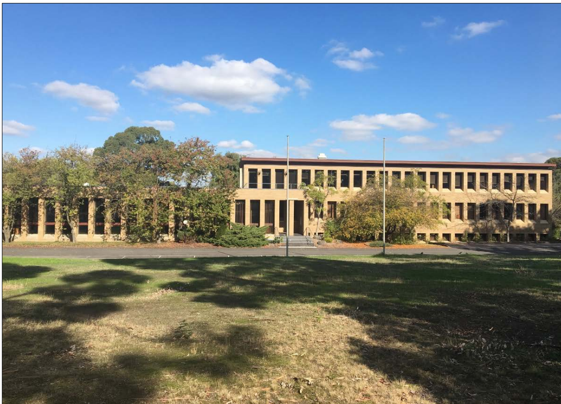
Figure 19 The front (north) elevation of the Administration Building.
