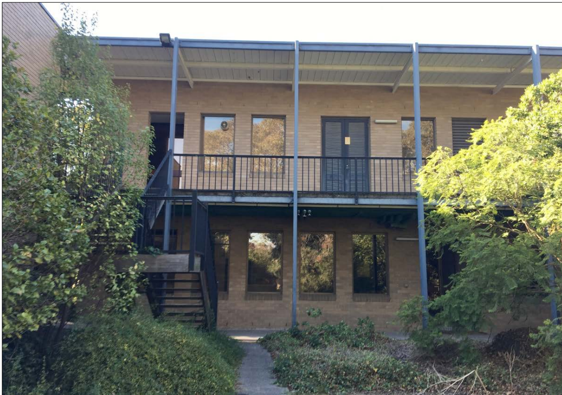
Figure 32 The west elevation of the Research Wing 2.
