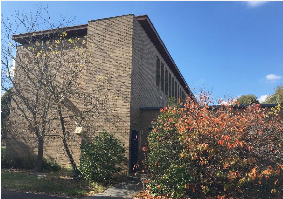
Figure 23 The west elevation of the Administration Building.
