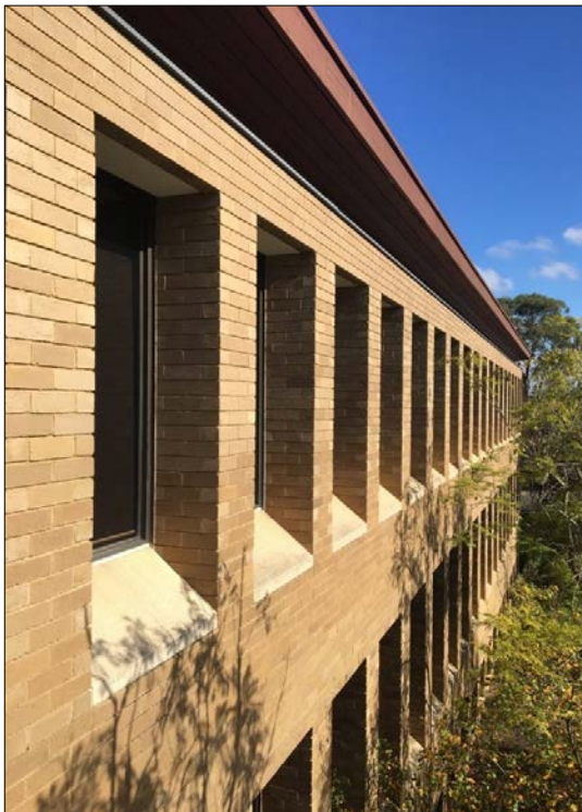
Figure 20 (left) Partial view of the north elevation of the Administration Building showing the deep window reveals and cornice like eaves detail.
