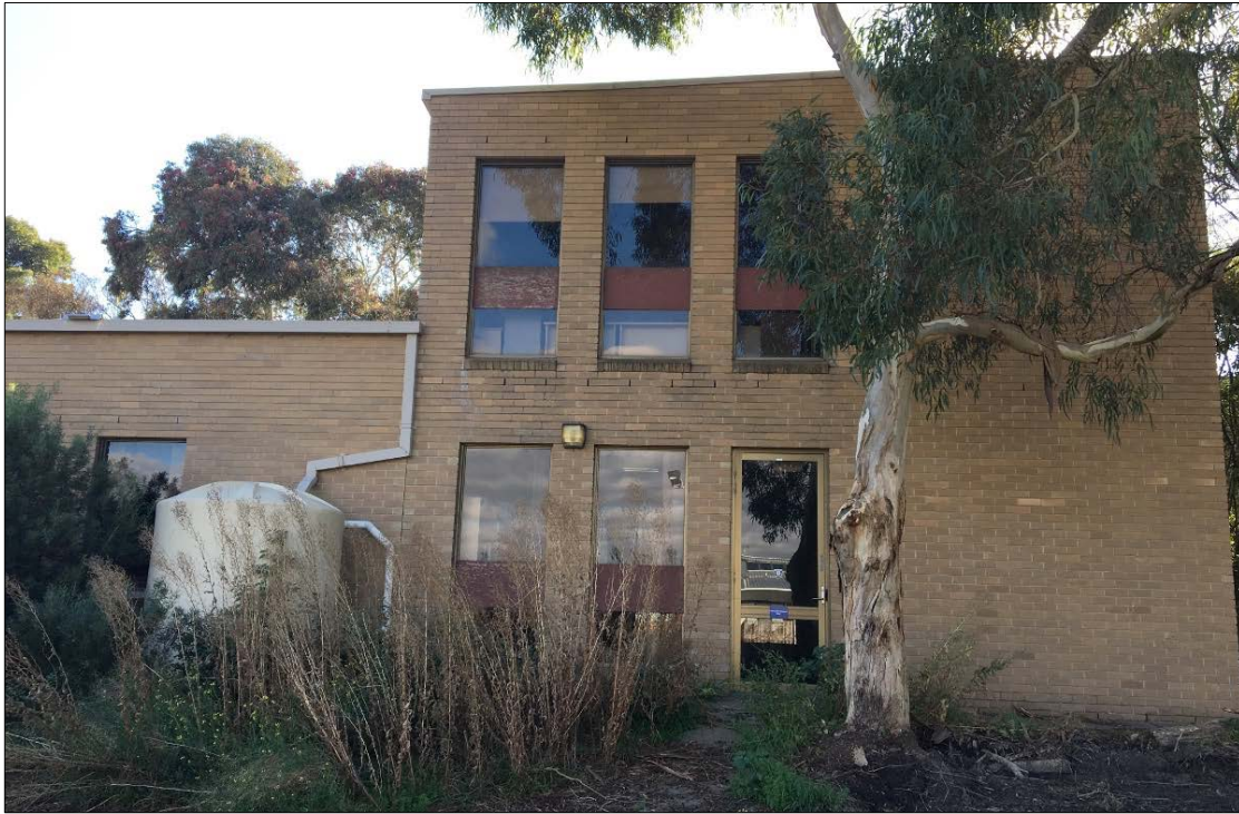
Figure 36 The south elevation of Research Wing 3.
