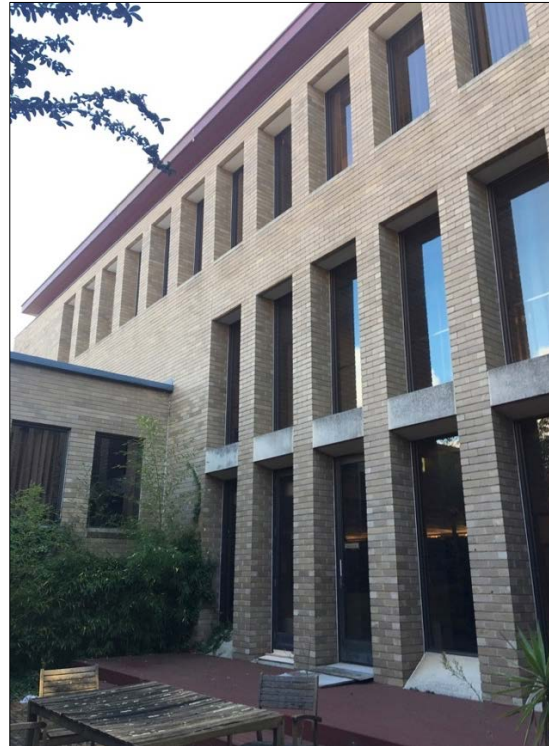
Figure 20 (left) Partial view of the north elevation of the Administration Building showing the deep window reveals and cornice like eaves detail.
