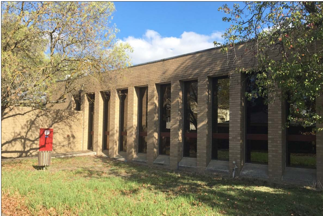
Figure 22 The east elevation (dining area).
