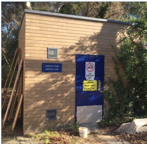
Figure 47 (left) Garden Maintenance Shed.
