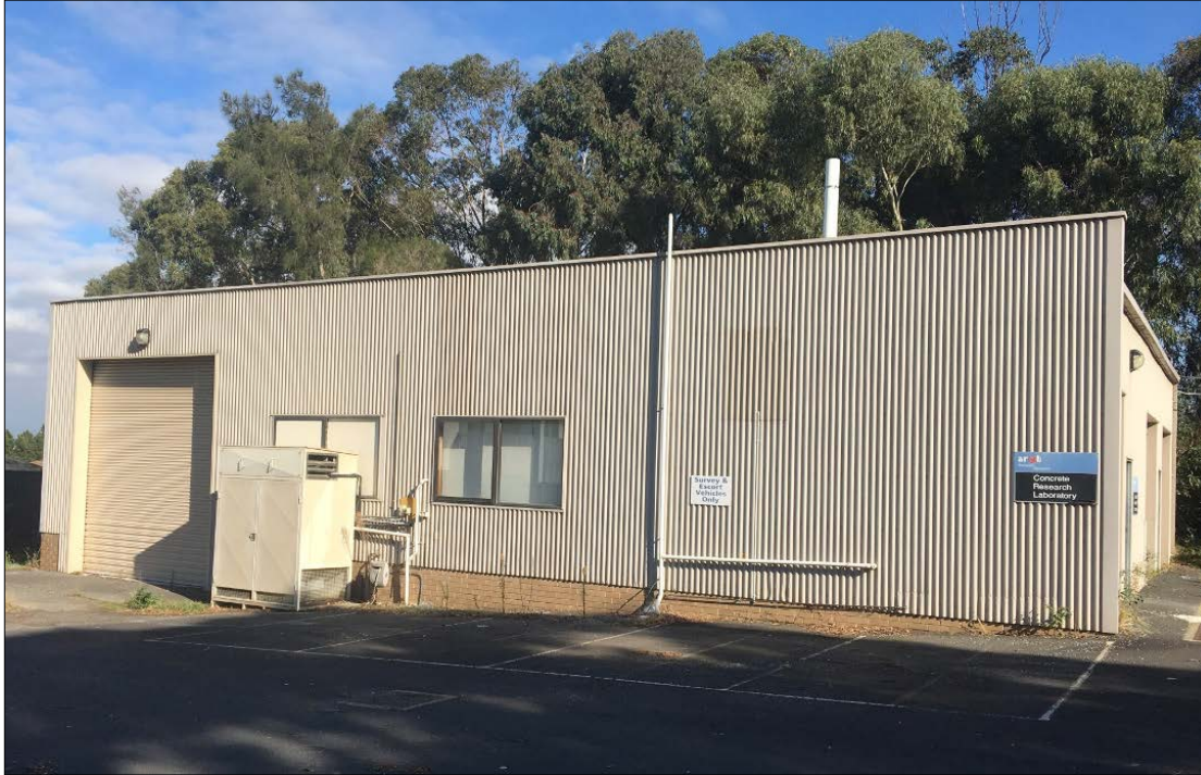
Figure 40 The Concrete Labs/HV workshop.
