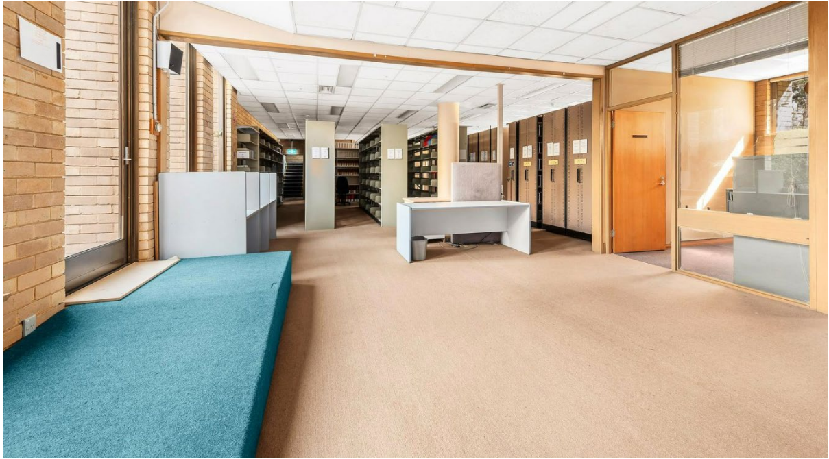
Figure 7 – Internal office arrangement pre fire
