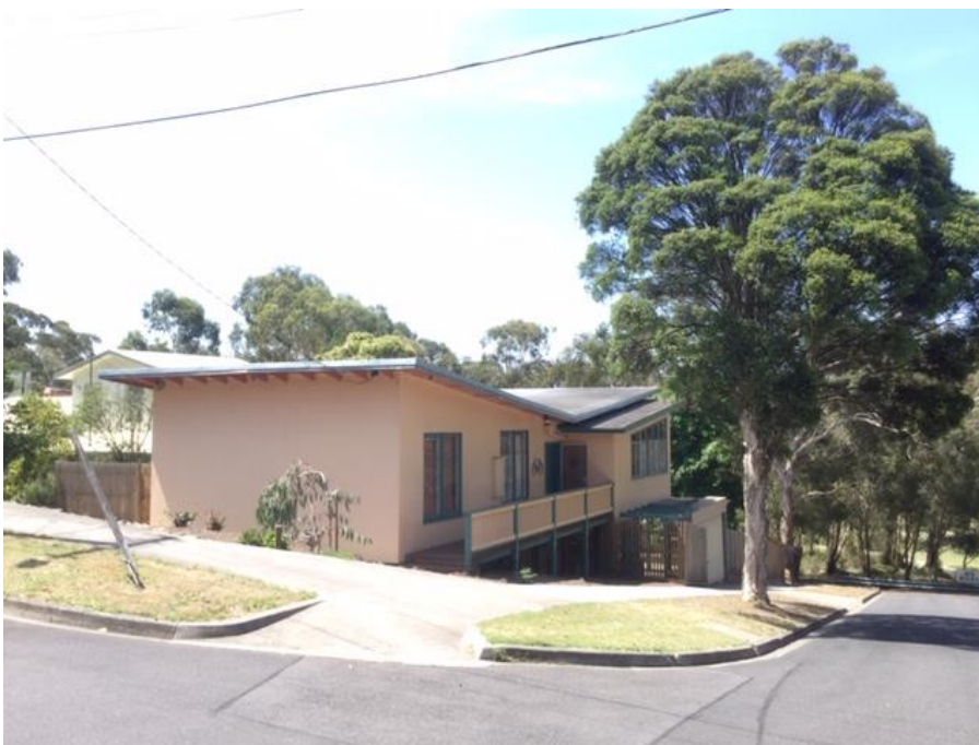
Plate 1 – 81 Orchard Crescent Mont Albert North, looking toward front aspect of property
