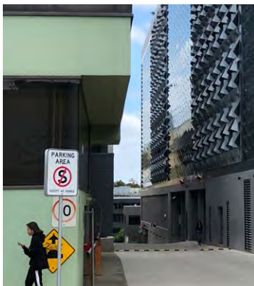
Figure 3 Higher density residential development with high-capacity car parks on Fairbank Lane.
