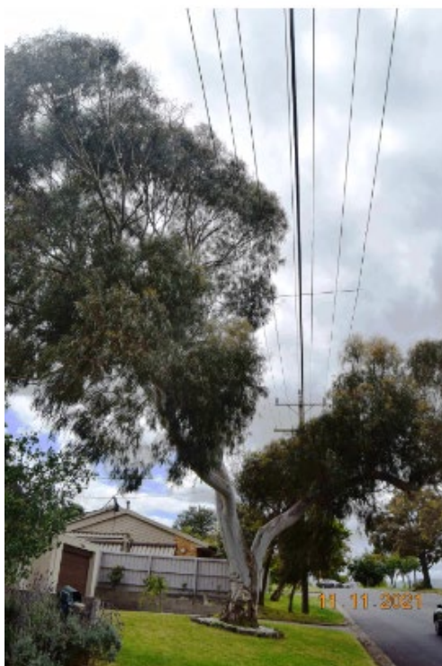
Figure 4 Street tree in conflict with electric lines
