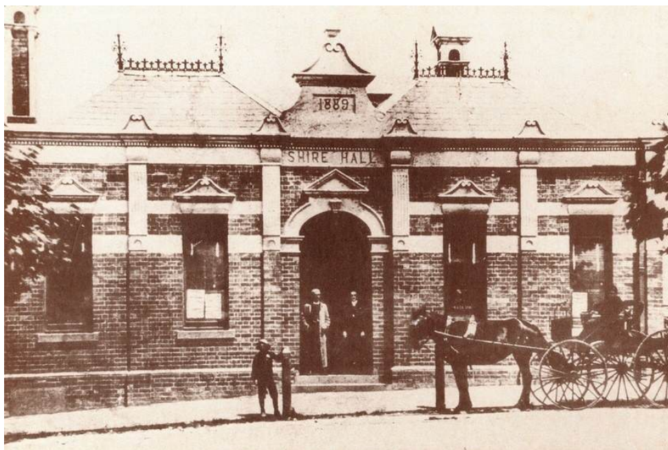
Figure 70. Nunawading Shire Hall, c1890 (Courtesy of the Whitehorse Historical Society Inc, no NP2817)
