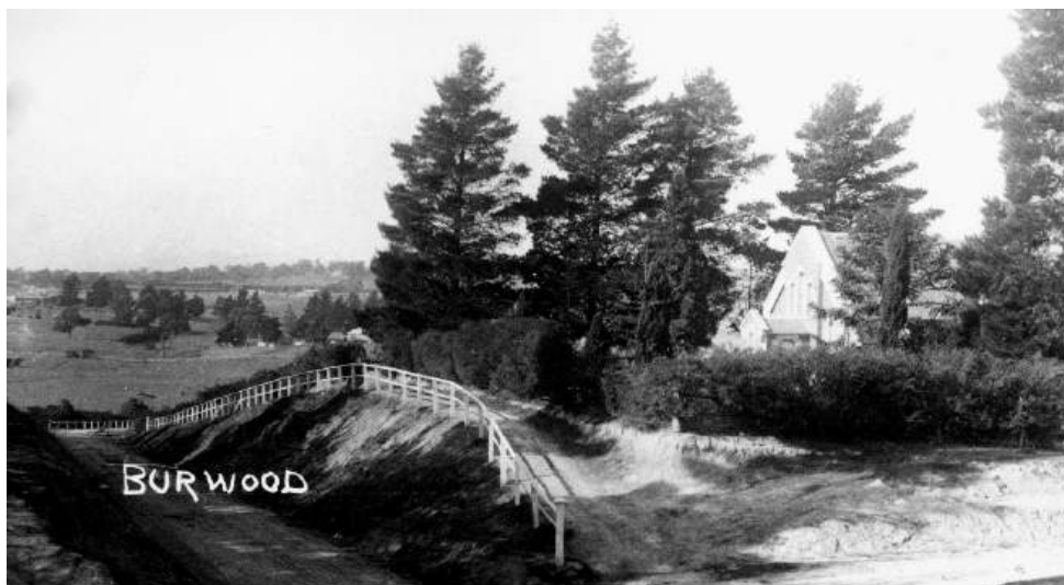
Figure 104. The Hoyts Skyline drive in cinema site at Burwood, c 1950s (Box Hill Historical Society, no B0928)
