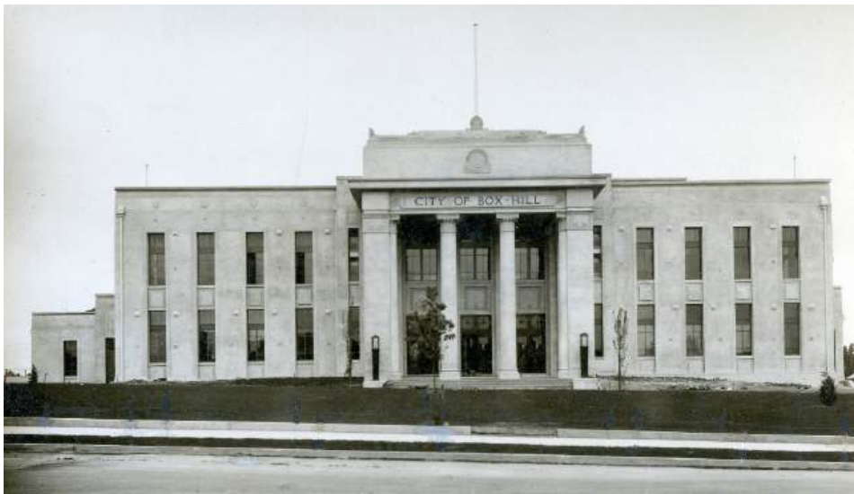
Figure 72. Box Hill Town Hall, c 1935 (Box Hill Historical Society, no 1025)
