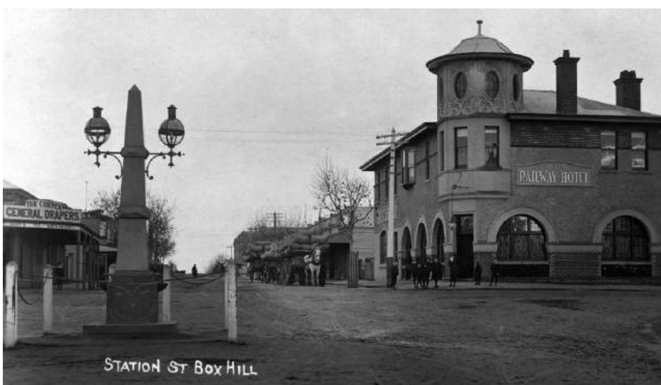
Figure 46. Looking south along Station Street, Box Hill, with the Railway Hotel to the right of the image (Box Hill Historical Society, no B9108)
