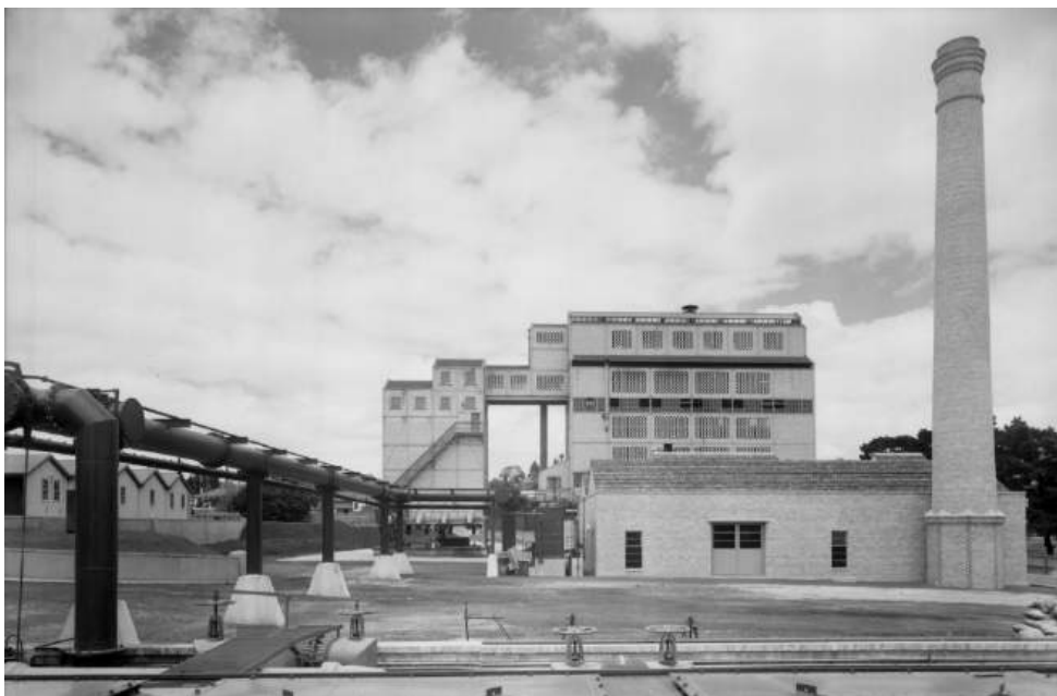
Figure 76. Colonial Gas Association gasworks, Box Hill, c 1945 (State Library of Victoria, ID 1642127)
