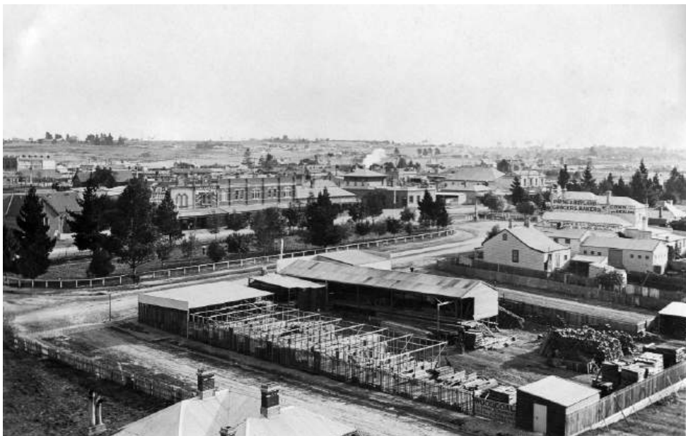
Figure 37. Looking south west across Whitehorse Road, Box Hill from the fire station tower, 1905 (Box Hill Historical Society, no B0915)
