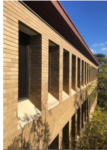
Figure 8. Detail of north elevation showing deep window reveals and recessed eaves. Source: Conservation Management Plan, Bryce Raworth & Associates Pty Ltd, Feb 2021.
