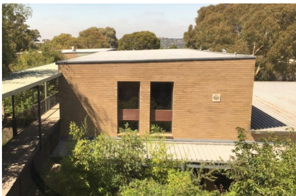
Figure 10. North elevation of Research Wing R1.
