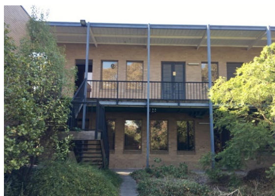
Figure 1. West Elevation of Research Wing R2.
