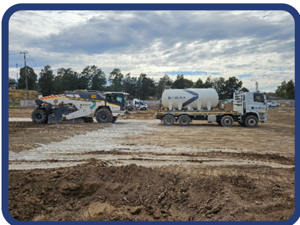
Stabilisation works in progress
