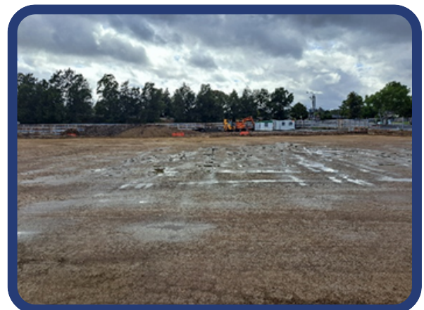
Stabilisation works completed
