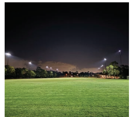
On demand lighting at Terrara Park – allowing greater utilisation throughout winter.
