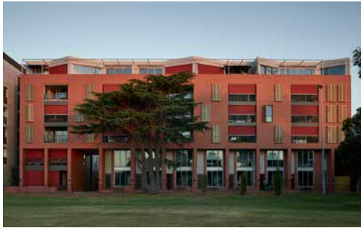
Housing fronting East Burwood Reserve. Balfe Park Lane, Nicholson Street | KTA
