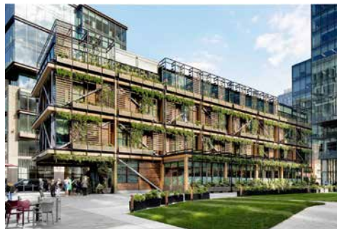
Commercial with hospitality fronting key walks | Hardman Square Pavilion, UK | Sheppard Robson
