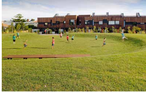
Townhouses fronting open space retention basin | Heller Street, Brunswick | Six Degrees Architects
