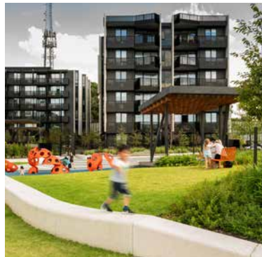
Housing fronting open space, Garden Apartments, Burwood Brickworks | Hayball
