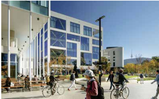
Office/education fronting public plazas. Marie Reay Teaching Centre, ANU | BVN & Lahznimmo Architects
