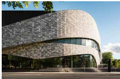
Conferencing gateway building. Te Pae Christchurch Convention Centre | Woods Bagot & Warren/Mahoney
