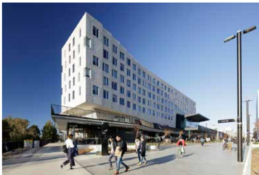
Student housing above commercial. Ferner Hall student accommodation, ANU | BVN
