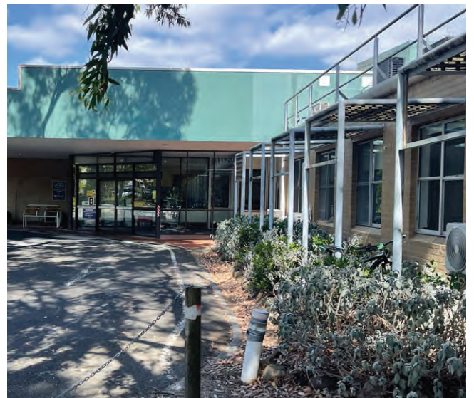
Figure 70 Peter James Centre building is beyond its reasonable life
