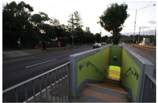
Figure 58 Deakin University / Burwood Highway tram stop underpass
