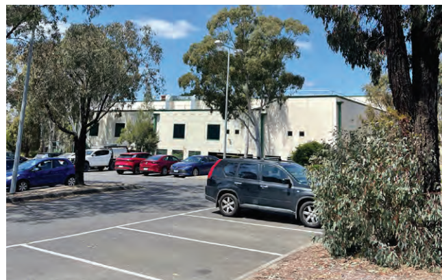
Figure 98 Inward facing buildings with tinted glazing
