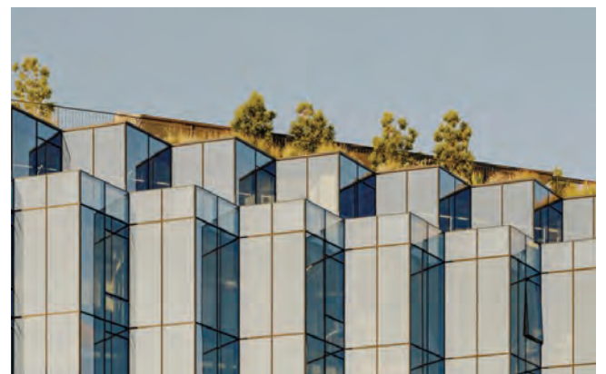
Figure 83 Green roofs and terraces can offer spaces for socialisation, collaboration and shared views — Encore, Cremorne | Fieldwork
