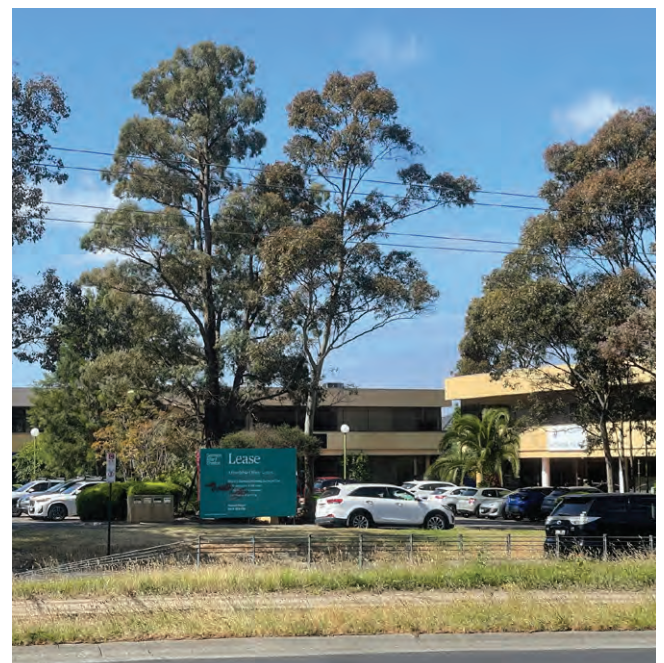
Figure 71 Mixed Use Zone north of Burwood Highway has the potential for redevelopment
