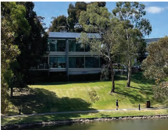
Figure 84 Overshadowing of Tally Ho Lake and open space is a key consideration in reviewing heights.
