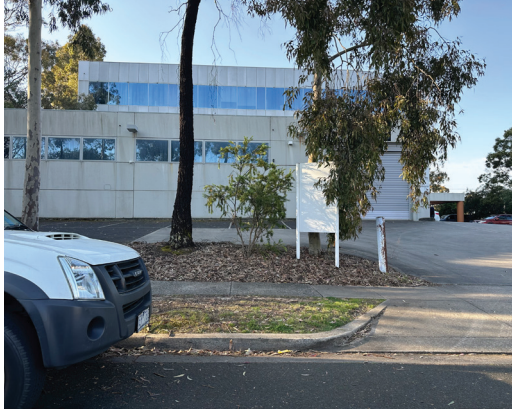
Ageing office park building with limited connection with the public realm
