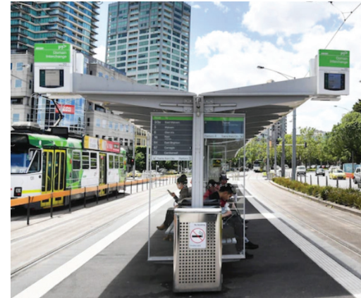
Accessible tram stop with extensive shelter, passenger information displays, Melbourne
